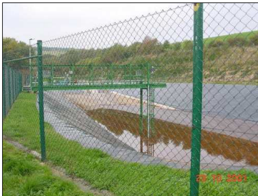
Figure 3.75: Water retention basin of German potash mine
