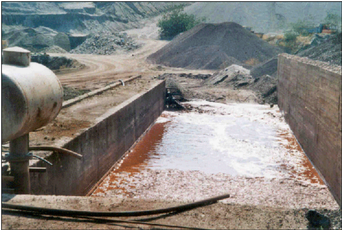
Figure 1.24: Example of a small tailings settling basin
