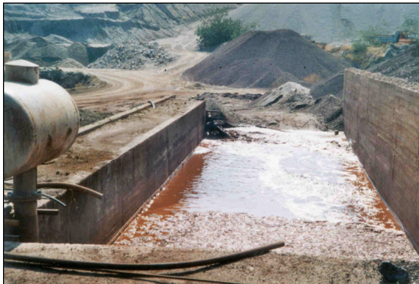
Figure 3.49: Dewatering of tailings in concrete basins [110, IGME, 2002]
