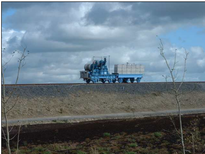
Figure 3.21: Electrically driven winch controlling the tailings distribution pipeline at the Lisheen TMF
